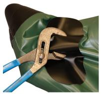
Place the material in the jaws of the channel lock pliers to protect the hull material. Once the body of is unscrewed from the base, pull the body from the opening and insert the replacement base. The opening is very tight, so you may have to pull on it hard.
