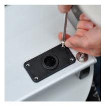
Place the rod holder mount into the mounting holes and secure with screws using a Phillips head screwdriver.
