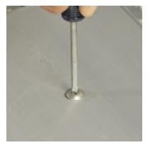
Tighten the screws on the underbars using a Phillips head screwdriver (not included). It is important to make sure that the aluminum boards and underbars are straight before fully tightening the screws.
