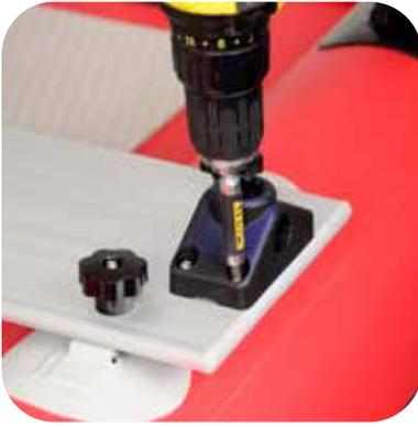
Attach Scotty rod mounts to the aluminum crossbenches with #6 x 1" truss head screws.
