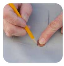
Using a pencil or ballpoint pen, trace the outline of the patch which should be large enough to overlap the damaged area by approximately 1/2". Angle the pen inward a bit so that the ink will be covered by the patch later.
